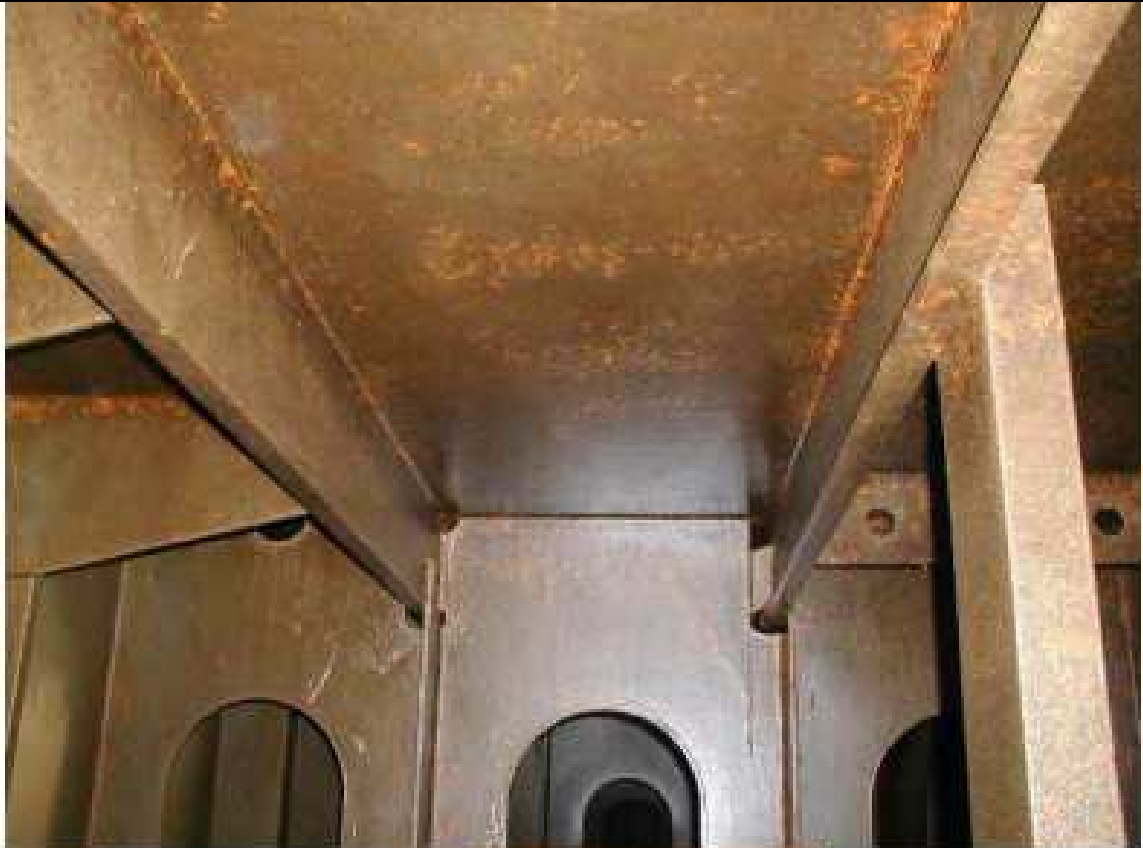
GOOD COATING CONDITION
