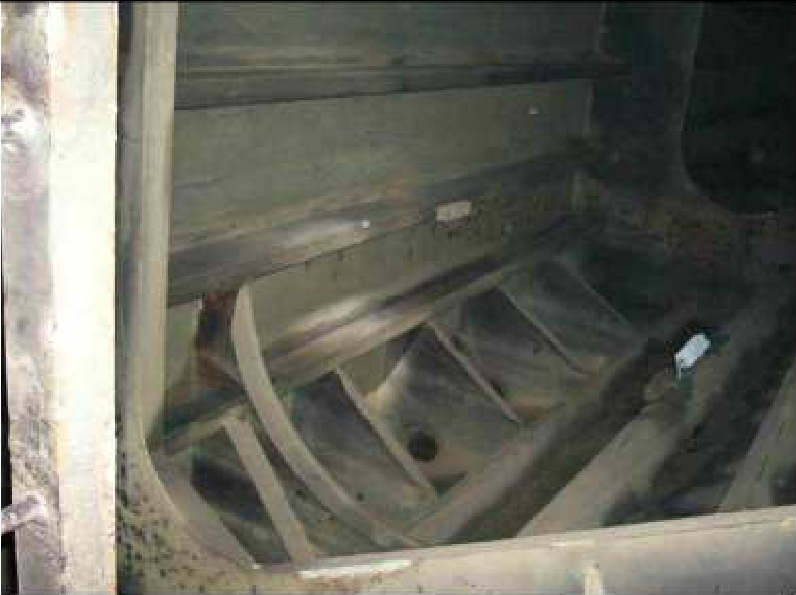
GOOD COATING CONDITION
