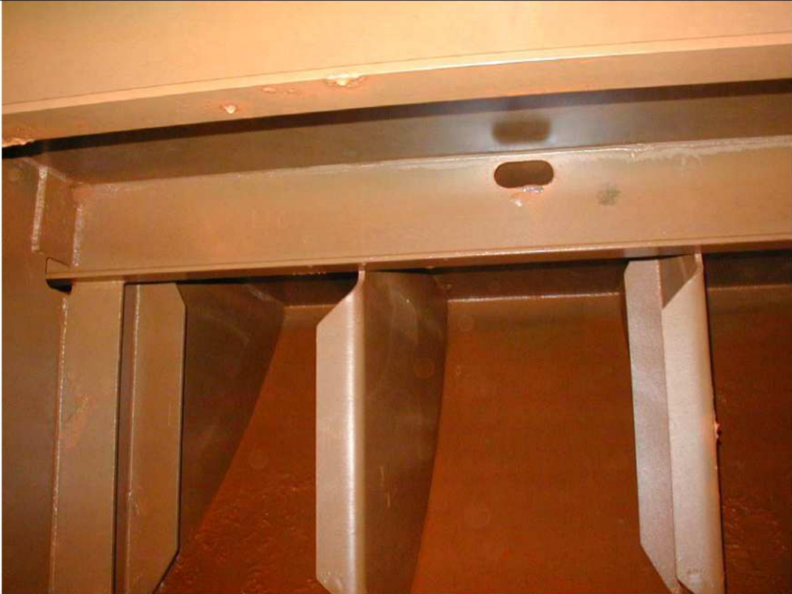
GOOD COATING CONDITION
