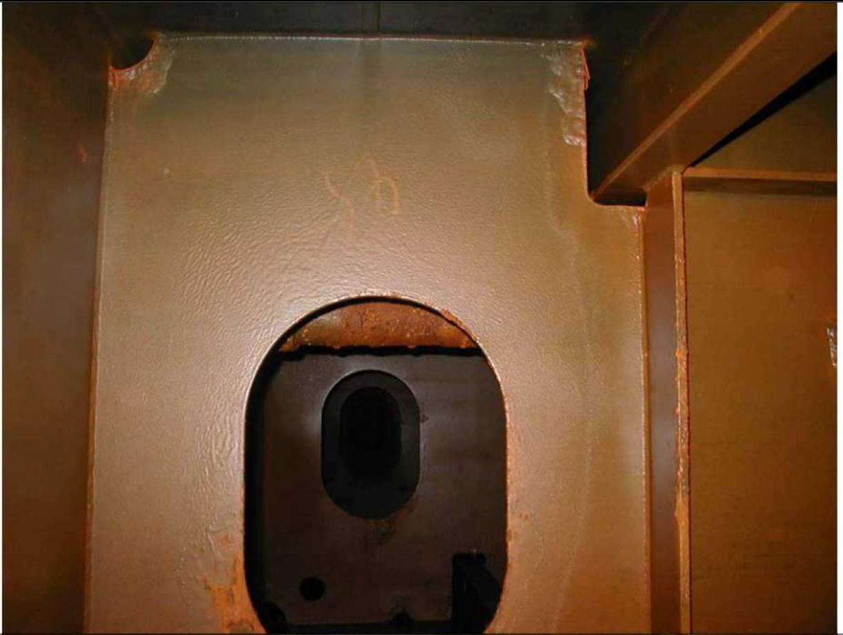
GOOD COATING CONDITION
